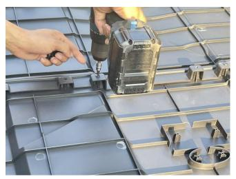
2. Take out the 4 limit brackets in the accessories package and fix them on the No. 2 and No. 3 interface with screws, and then fix the remaining mounting holes with screws. As shown in picture:
