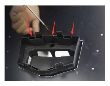
10. Clamp the top cover of the vent ,and then install the vent onto the aluminum roof by screws.
