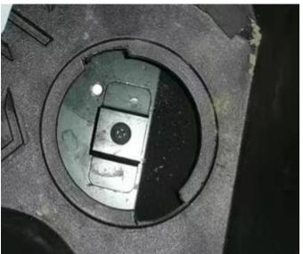
3. Screw the drain hole cover into the hole and complete the installation. As shown in picture:
