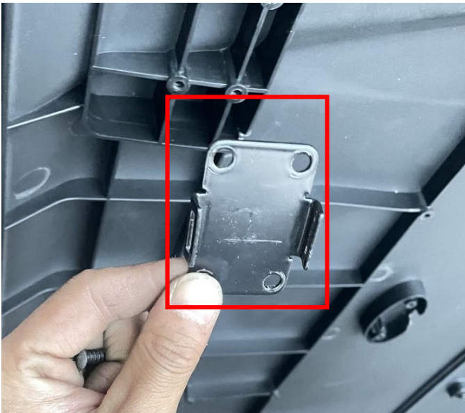
2. Fix the two iron square mounting brackets in the package to the roof with self-tapping screws. As the picture shows:
