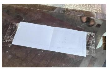
4. Use a 3mm drill bit to drill holes according to the positions of the screw holes on the locator sheet, and then use a cutter to cut the holes according to the locator sheet.
